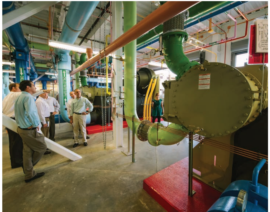
University community members view the Central Energy Plant's color-coded piping and equipment that provide chilled water for air-conditioning throughout campus.
