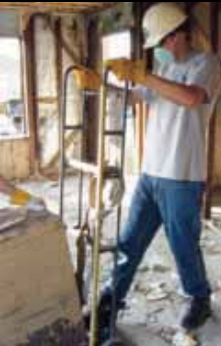
Patrick Godfrey at work in one of the four homes the LAKO team helped clear of debris
